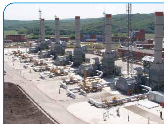
Kasimovskoye UGSF is one of the 24 gas storage facilities operated in the Russian Federation, 7 of them being located in water-bearing structures and 17 at the exhausted fields. In 2005, a total of 46.3 bcm of gas was pumped into the gas storage facilities located in Russia and a total of 42.8 bcm was withdrawn. The pumping and withdrawal were done using 17 compressor stations and 235 gas pumping units with a total installed capacity of 1,021.7 thousand kW.
